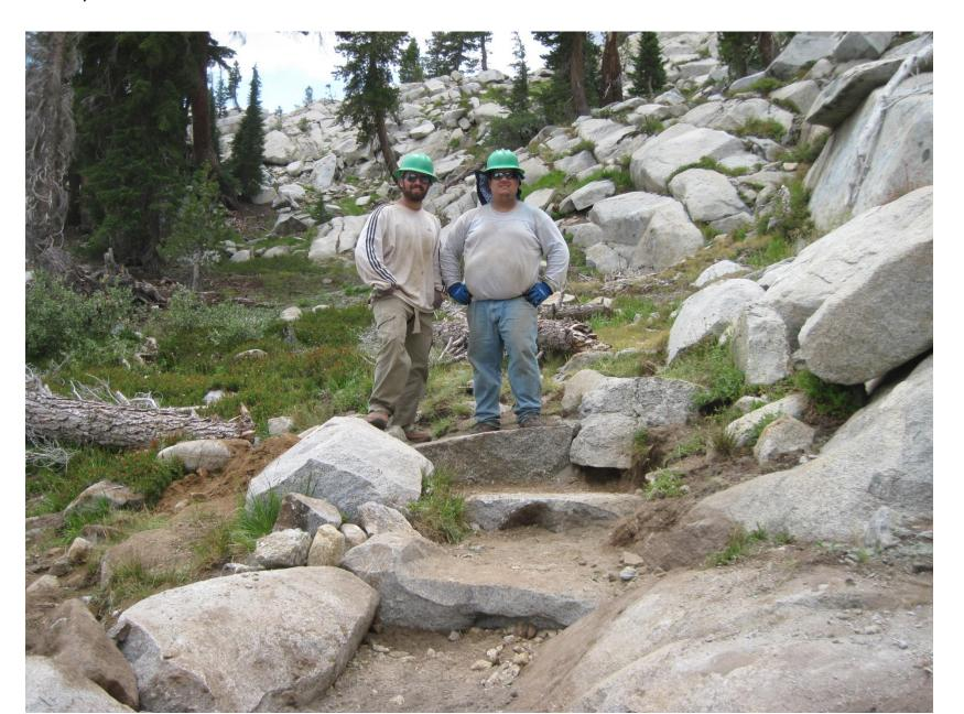
Repair heavily eroded gully in trail by: rebuilding switchback and placing 1 step with associated anchor rocks, walls and crush fill.
