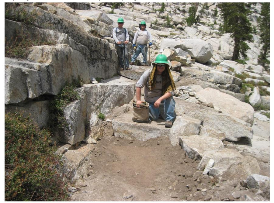
Repair rutted trail, rebuild switchback, place step, anchors, wall and crush fill
