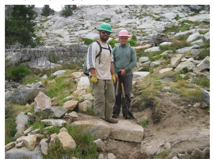
Repair deeply eroded switchback: Rebuild rock walls, place two steps, place crush fill
