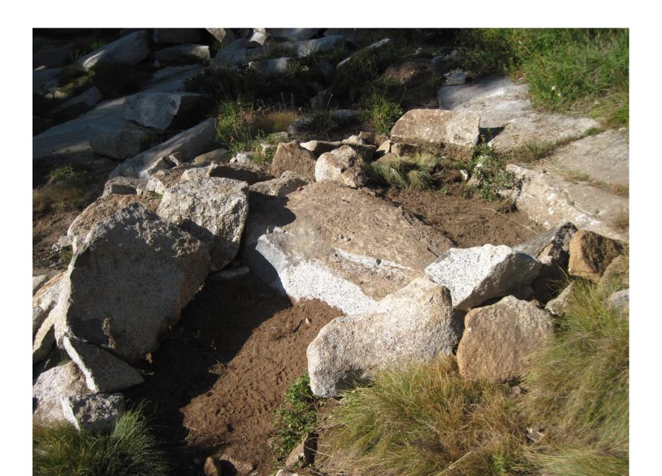
Repair heavily eroded gully in trail by: building and placing 3 steps with associated anchor rocks, wall and crush fill.
