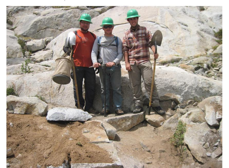
Repair deeply eroded trail and place substantial rock water bar and anchor rocks
