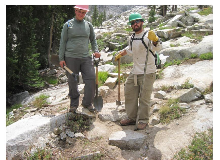
Repair heavily eroded gully in trail. Place 2 steps with associated anchor rocks, walls and crush fill.
