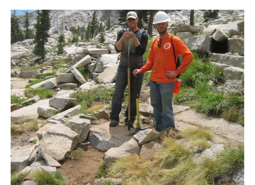
Repair heavily eroded gully in trail. Place 1 step with associated anchor rocks, walls and crush fill.
