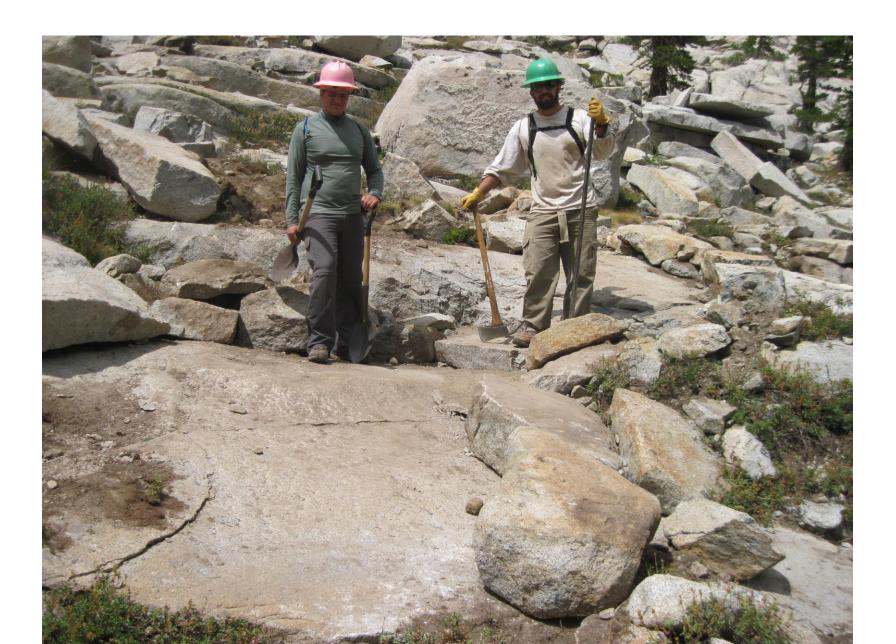
Repair heavily eroded gully in trail. Place 2 steps with associated anchor rocks, walls and crush fill.
